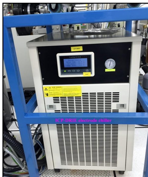
Fig.7 ICP-DRIE electrode cooling chiller
