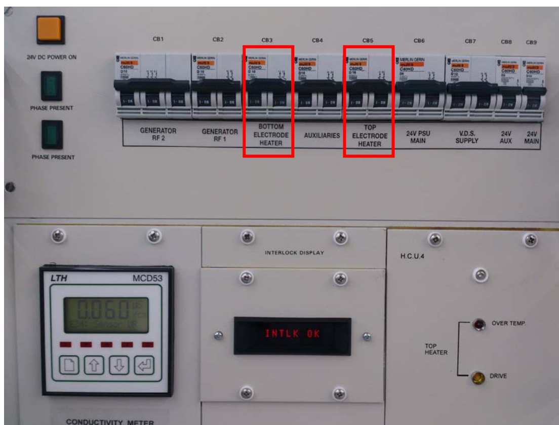
Fig 2: Position of the circuit breakers of top and bottom electrode heater
